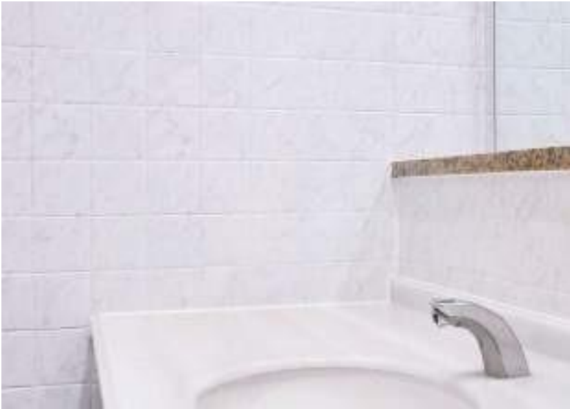
Restroom refurbishment / ST-024TIL
